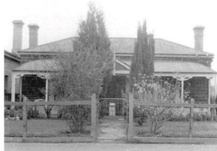
The house purchased by CIWA in 1953 in Carrington Street, Adelaide. In 1957 it was demolished and a hall was built in its place.
